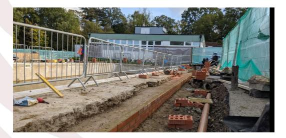
To date, pool building work has included all demolitions, diversion of existing services and utilities to the pool site, excavation and concreting of all foundations. We are delighted that work on our pool continues - this holiday, work was underway on the construction of the external walls. Although these have been built in fair face concrete blocks, the first courses (potentially subject to dampness) are being constructed in engineering bricks.
