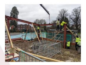
.... BUT by far the most exciting development has to be the swimming pool! Despite the weather, the steels have all been delivered and their erection is now fully underway.
